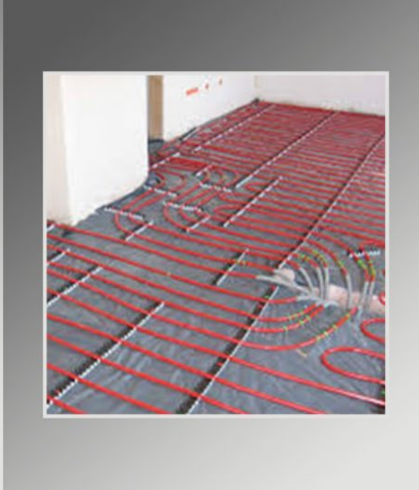
Underfloor heating 30 - 35°C
