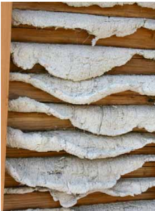
This image shows haired lime mortar pushed through a lath wall producing a key
