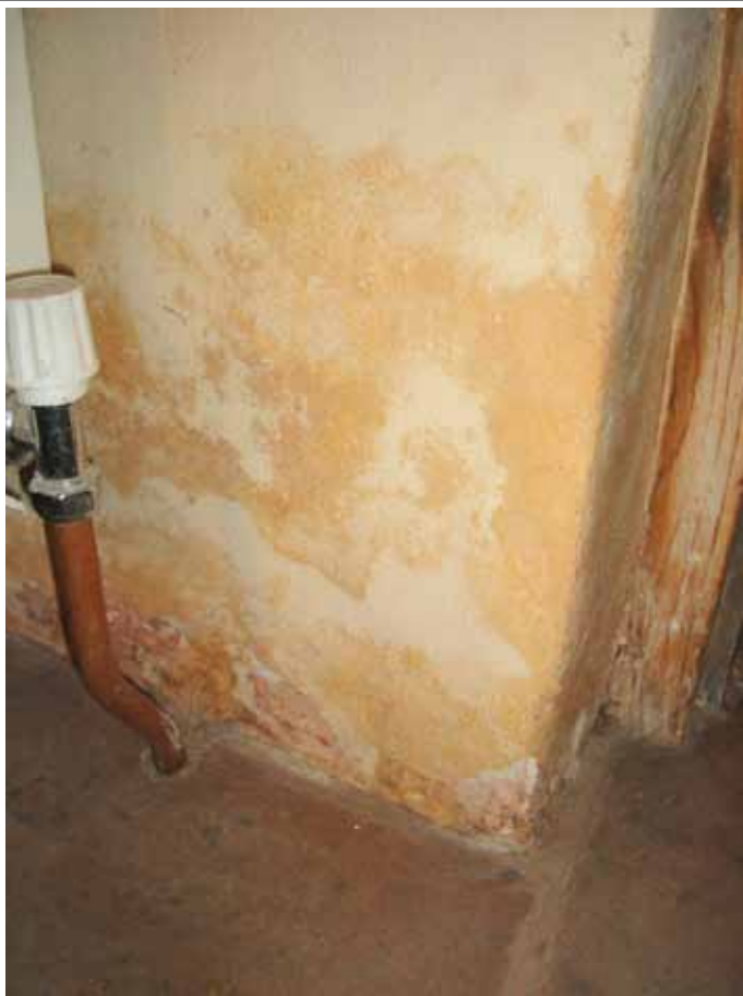
Typical problems that may occur when the floor has been sealed and the outside render is a hard cement covered with a modern non-breathing masonry paint.
