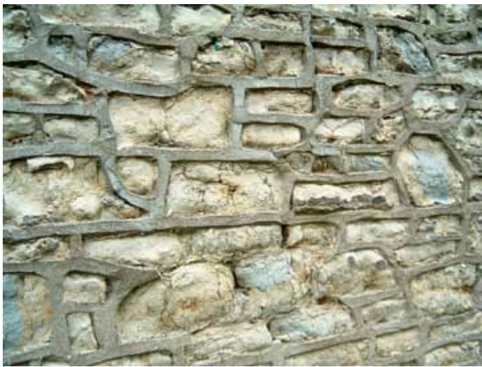
Damage caused by inappropriate, hard cement pointing
