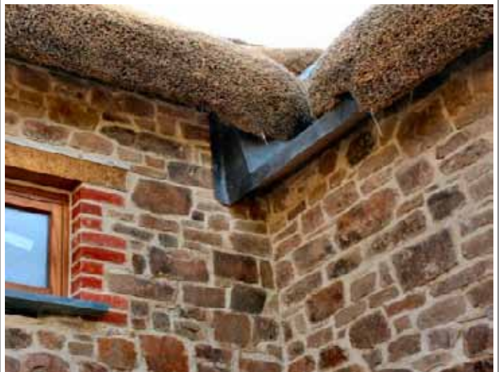
The correct way to point a stone rubble wall
